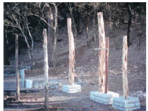
New posts for Interpretive signs
