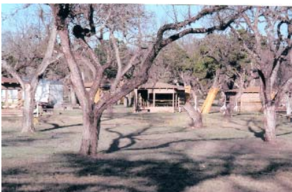
River Crossing shelter under repair
