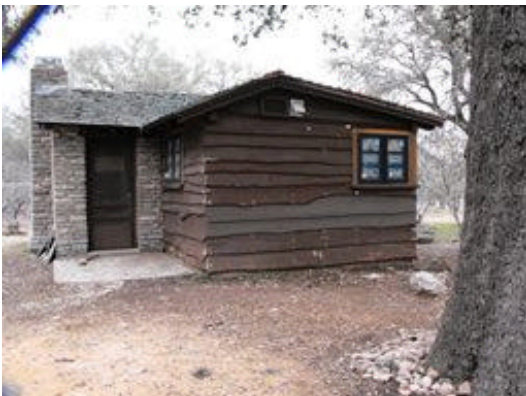
Cabin 1, Garner State Park, under renovation - Dec. 2011
